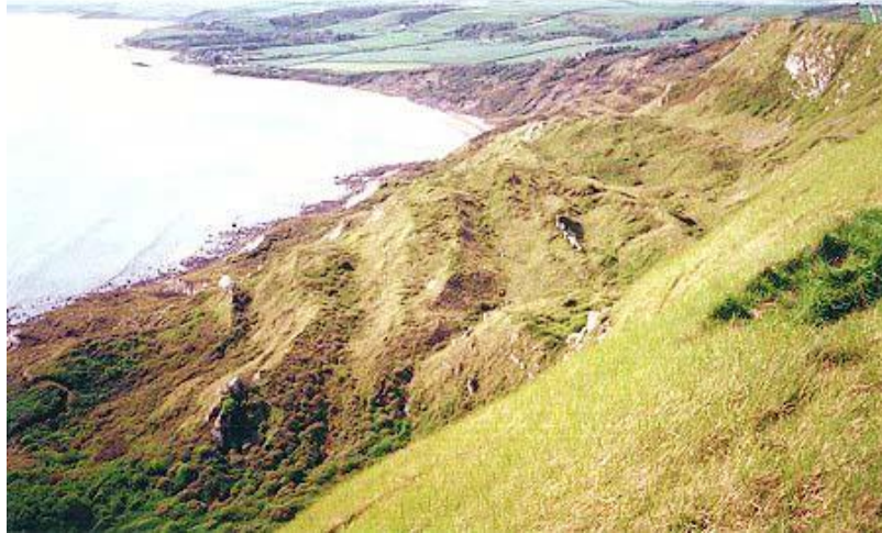
Fig. 7: Photograph of a slump (rotational slide)
