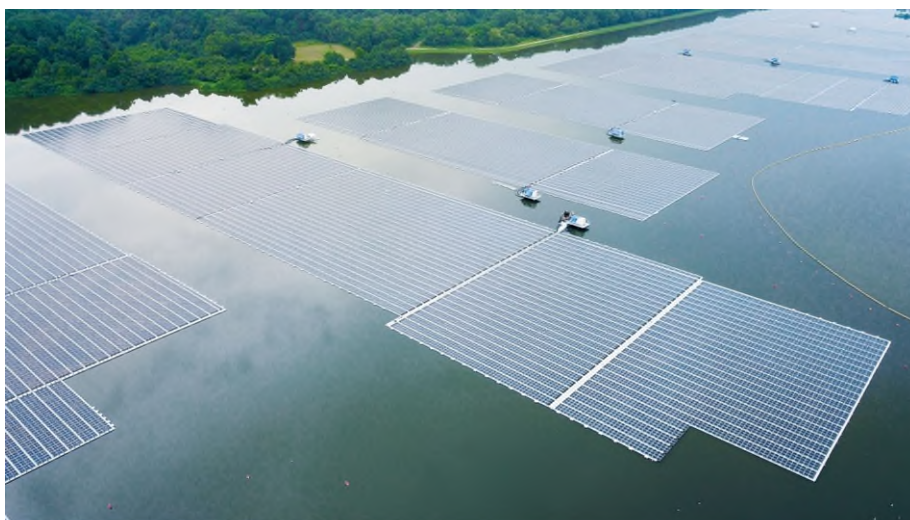
Aerial view of Sembcorp Tengeh Floating Solar Farm, Singapore.
